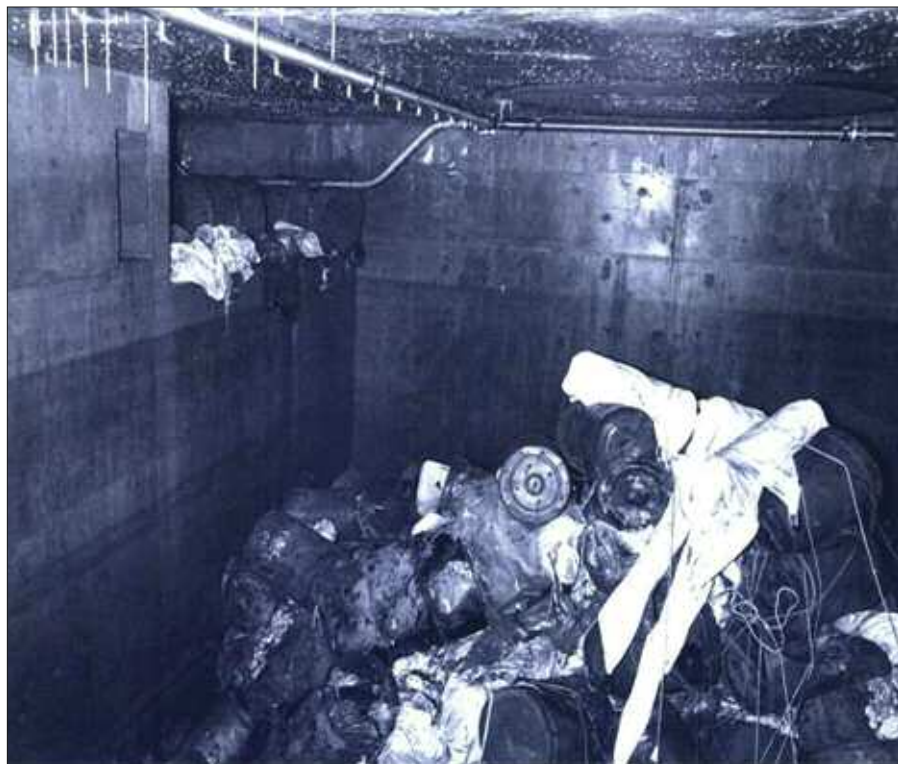
Accumulated waste inside the silo in the 1980s (Photo: DSRL/NDA)
